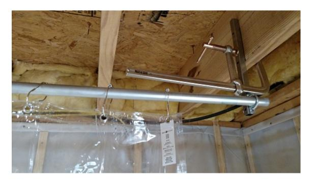
F clamp used to temporary hold tubing until secured with lag bolt
